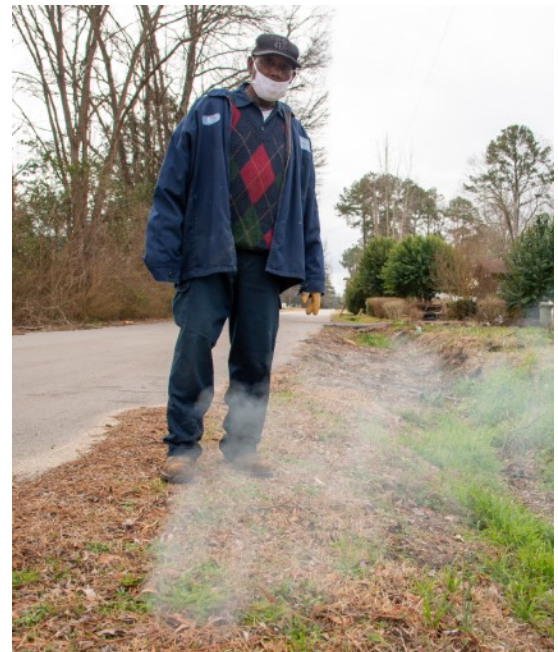
Maintenance Employee James McMillian investigating where the possible leaks into the sewer system. Photo by Michael Dantzler
